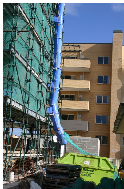
Figure 2.15.2 - Example of management of construction waste.
