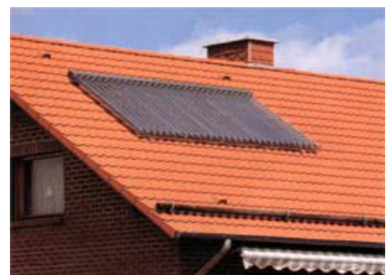
Figure 2.4.2 - Solar hot water panels facing north.
