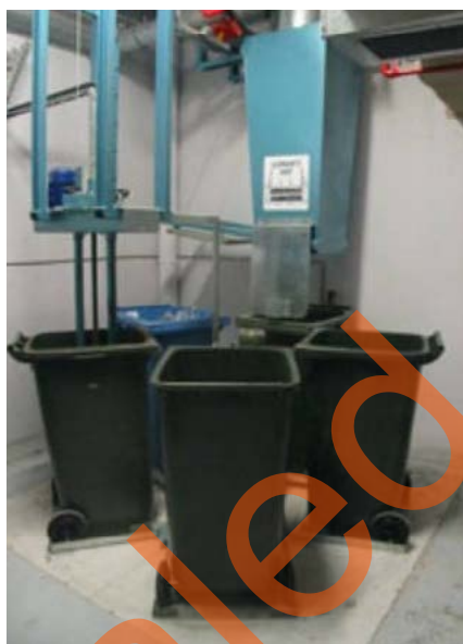
Figure 5.4.9 Example of waste chute within a residential apartment building.
