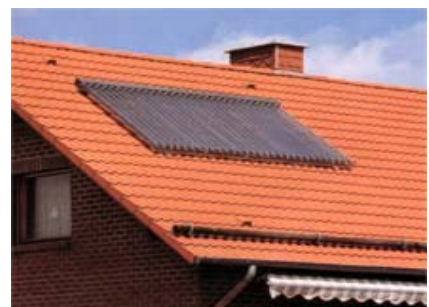
Figure 2.4.2 - Solar hot water panels facing north.
