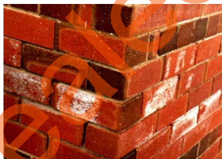
Figure 2.14.1 - Salt damage in the brickwork of surrounding properties identifies a possible salinity problem in the area.
