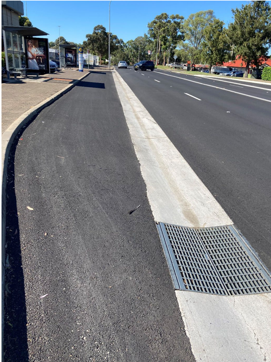
Dish Drain at Brookfield Road, Minto
