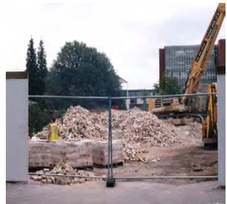
Figure 2.9.1 - Demolition waste materials separated and stored on-site until they are safely removed for reuse, recycling or disposal.
