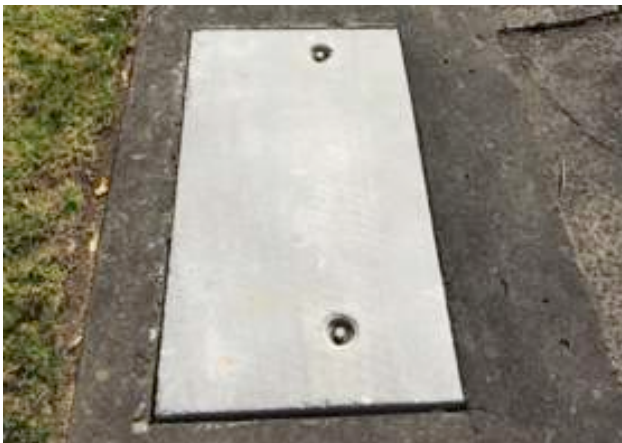
Reconstructed stormwater pit at Hobart Avenue, Campbelltown
