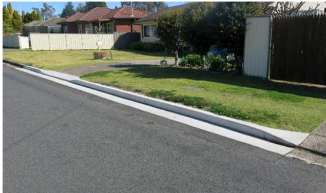
Kerb and gutter along with layback at Paterson Street, Campbelltown
