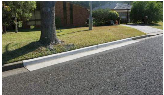
Reconstructed kerb and gutter at Endeavour Street, Ruse
