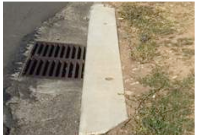
Reconstructed stormwater lintel at Pembury Road, Minto
