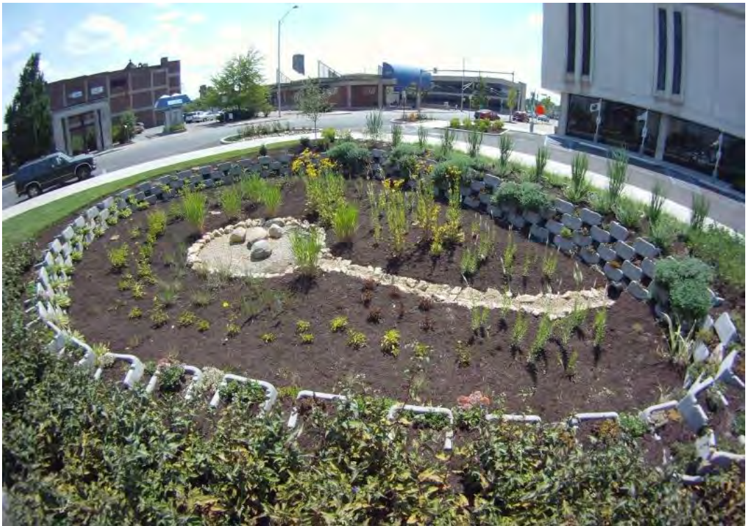
Figure 6: Photo of Typical Bioretention Basin
