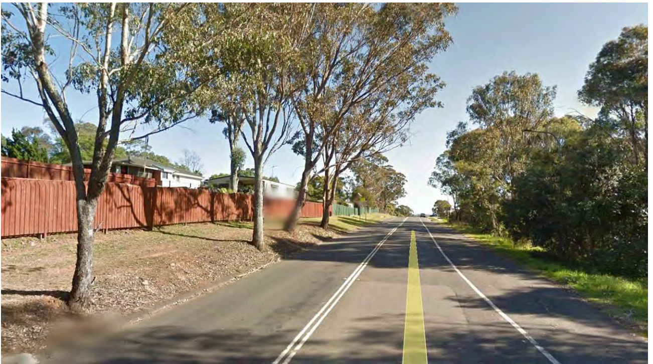
Photograph 5 – Westmoreland Road in the vicinity of the site.
