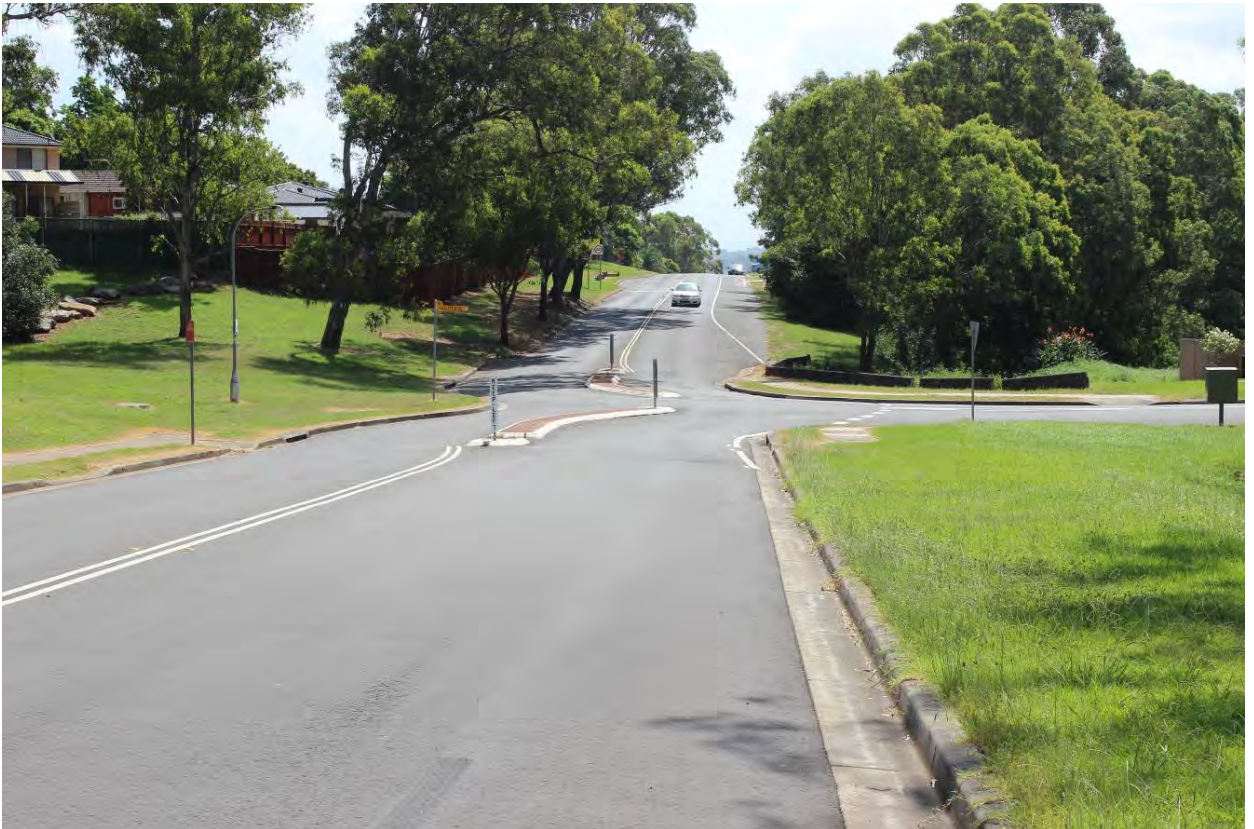
Photograph 5 – Westmoreland Road in the vicinity of the site.
