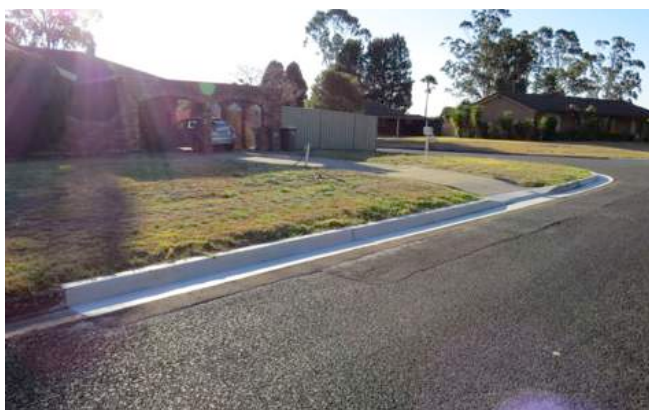
Kerb and gutter along with layback at Dandenong Crescent, Ruse after reconstruction
