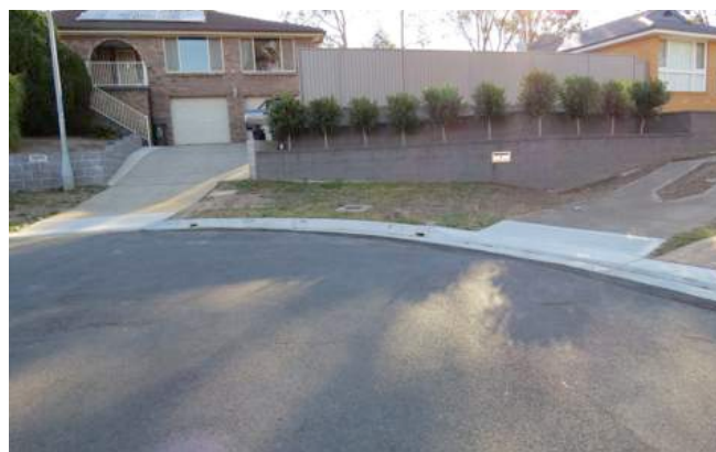
Kerb and gutter along with layback at Yulunga Place, Bradbury after reconstruction
