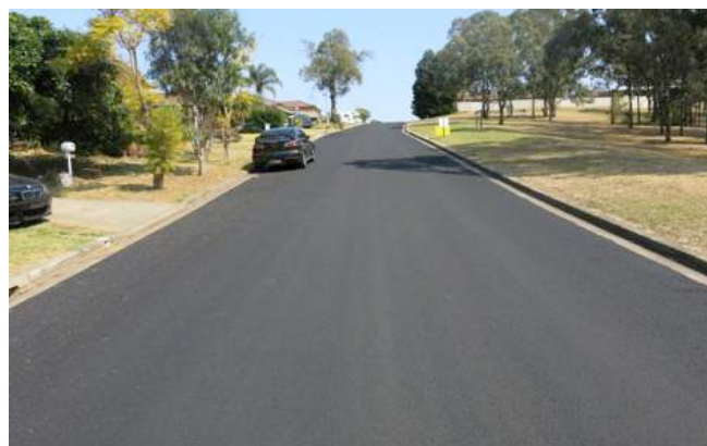
Lockheed Street, Raby after microsurfacing
