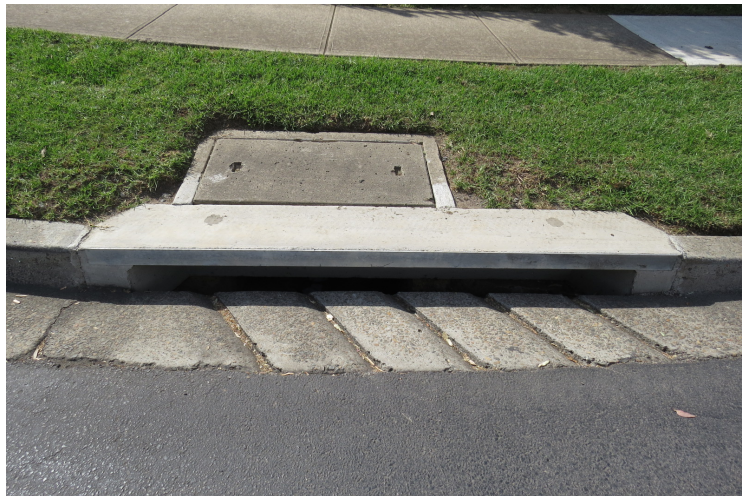
(Stormwater pit lintel replacement at York Place, Ingleburn)
