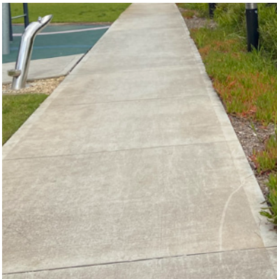
Concrete footpath- Broom finish to match existing
