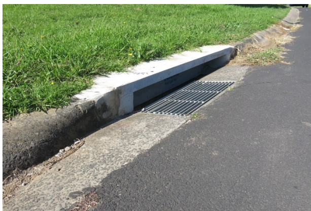
Stormwater pit lintel replacement at Parnell Close, Minto
