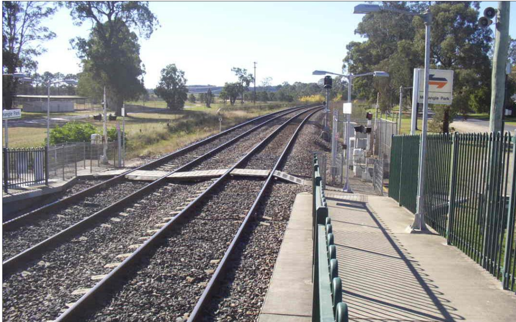
Figure 5.5 – Menangle Park Station
