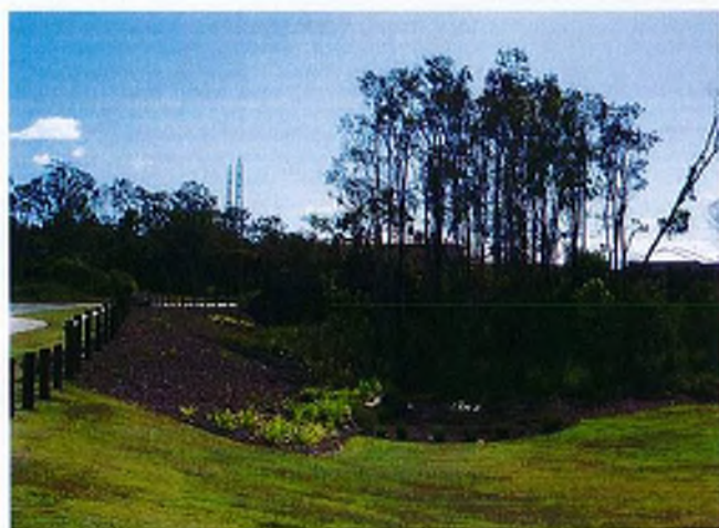
Figure 7.8 Vegetated bioretention system as part of a detention basin
