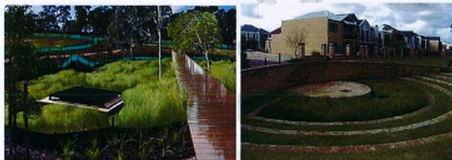
Figure 7.11 Detention basins may include paths, board walks, wetland pools, varied batter slopes and basin floor elevations and other landscape elements and variety of vegetation types to create interesting public open spaces.
