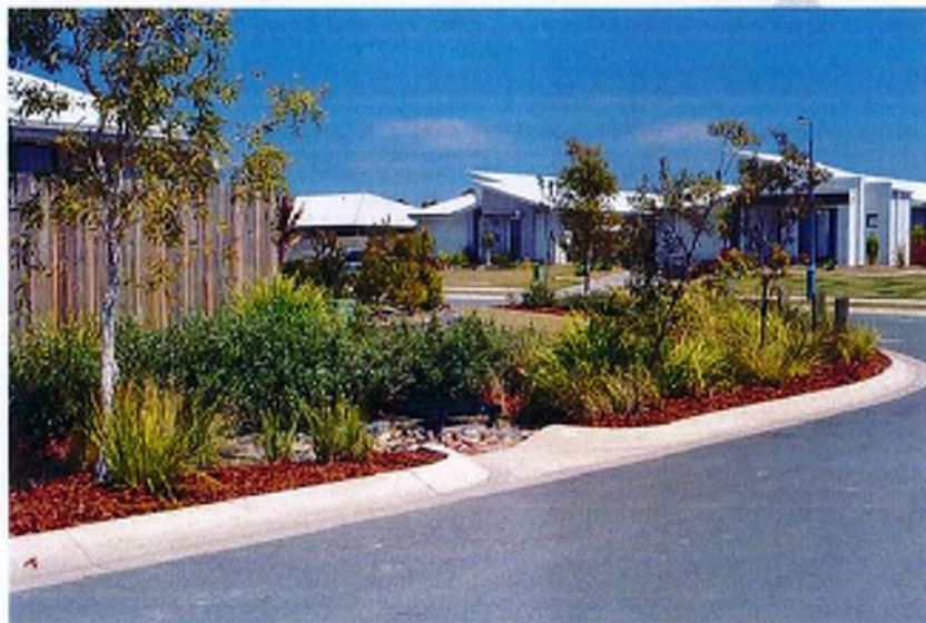
Figure 7.15: Bioretention in the street verge within residential estate (Photo A Cook, AECOM)
