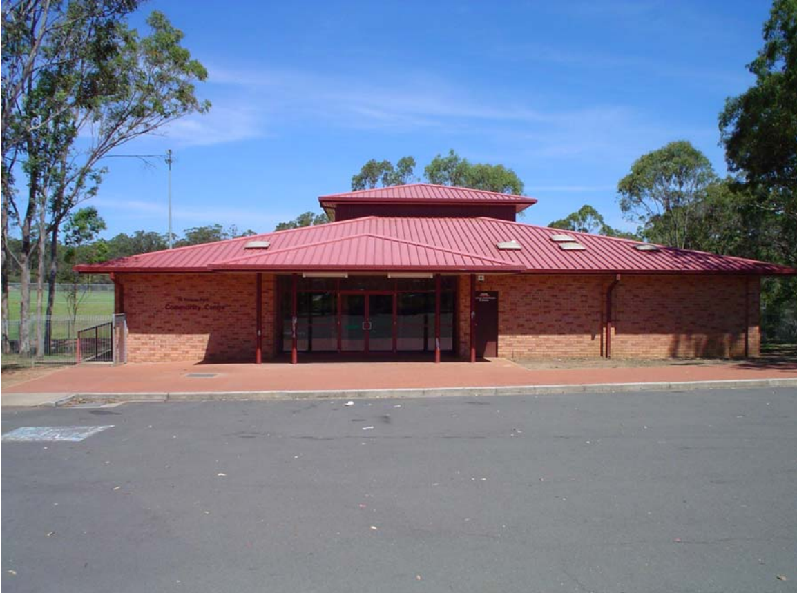
Figure 3: St Helen's Park Community Centre
