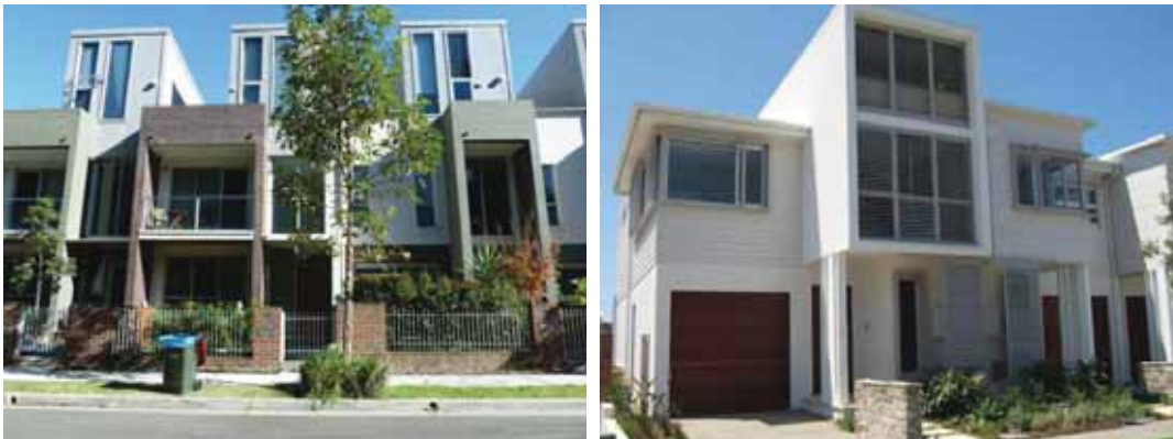
Examples of 3rd storey element providing good streetscape articulation
