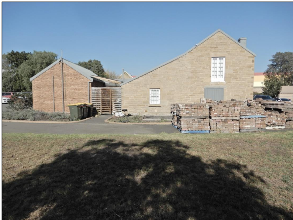
Figure 8: Warby's Stables (Source: Lucas Stapleton Johnson Heritage Report)
