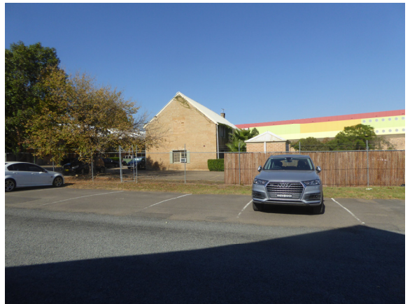
Figure 10: East elevation of Warby Barn with DFO building in background, as seen from the Warby Stables site to the east.
