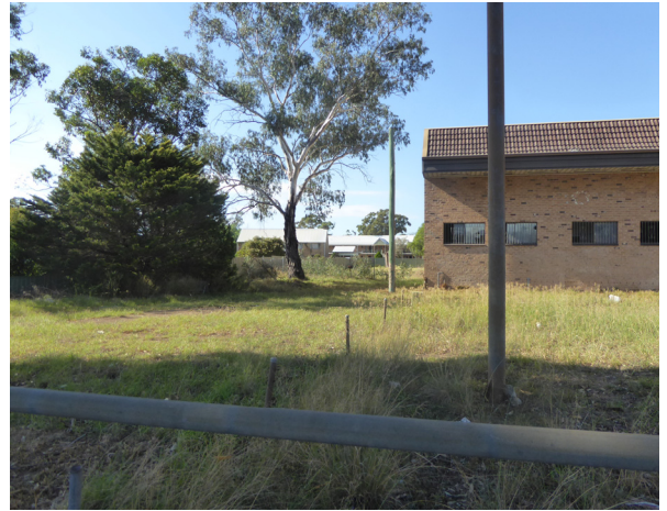
Figure 14: View of Warby Stables as seen from the subject property looking east across No. 24 Queen Street.
