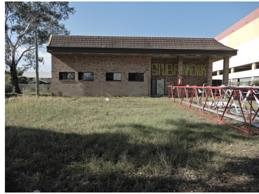
Figure 4: Former ten pin bowling building at No. 24 Queen Street
