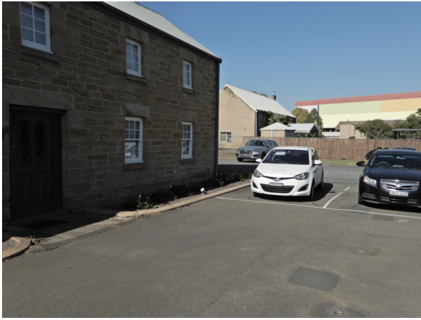
Figure 13: Front elevation of Warby Stables, with Warby Barn behind and the DFO on the subject property as backdrop.
