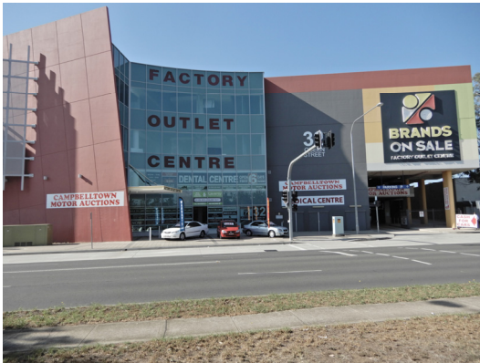
Figure 3: The DFO at No. 32 Queen Street
