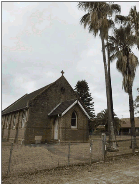
Figure 3: St James Anglican Church 2018
