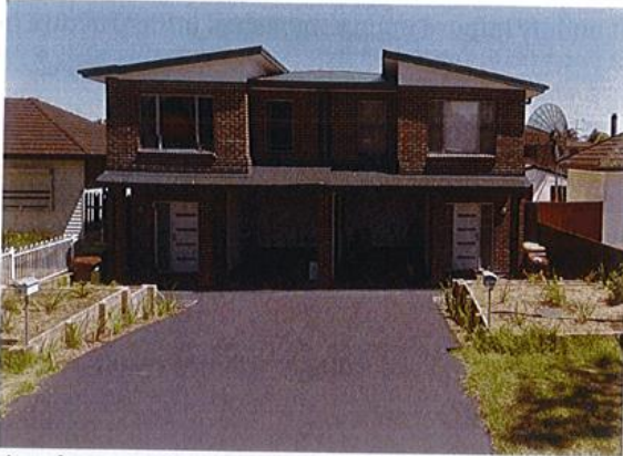
Another example of semi-detached dwellings at No. 25 and 25A Brenda Street (640/2014/CDCPDW).
