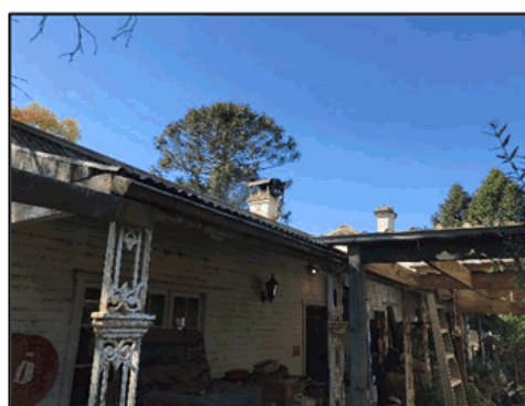
Figure 15. western elevation of subject site.
