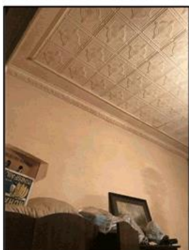
Figure 31. View of non-original yet contributory pressed metal ceiling in first bedroom
