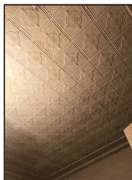
Figure 32. View of non-original yet contributory pressed metal ceiling in first bedroom
