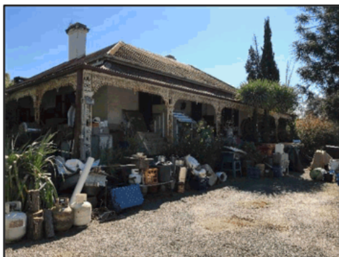
Figure 14. Subject site facing the front facade
