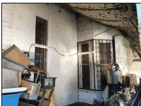
Figure 16. Western elevation of subject site. Note non-original bay window
