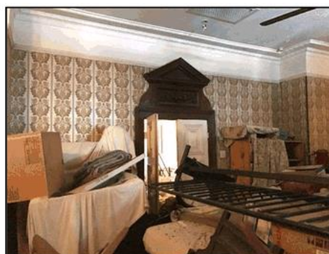
Figure 28. View of modified internal front room.
