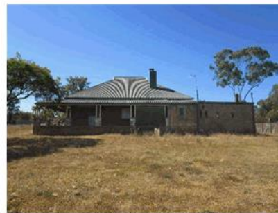
Figure 24: The north-west façade of the building.
