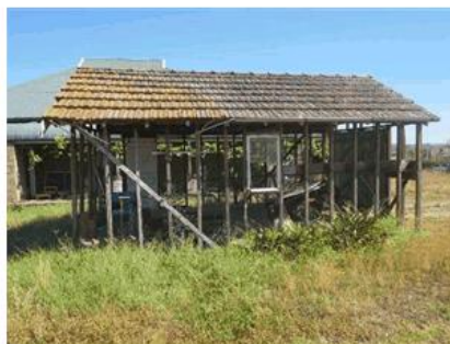
Figure 31: The garage structure to the south-east of the house.
