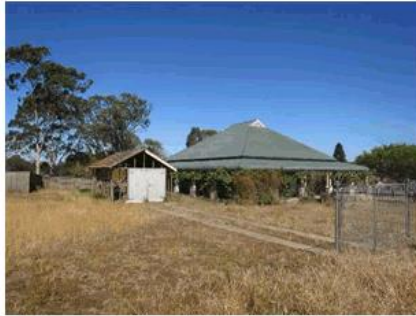
Figure 15: View of the subject site from Oxford Road, facing west.
