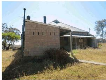
Figure 29: View of the rear wing of Woodcrest, facing north-east.
