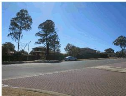
Figure 19: Surrounding residential area on Oxford Road, opposite the subject site, facing south-east.
