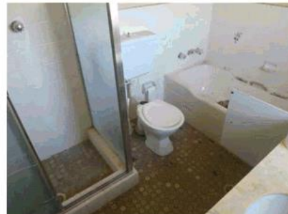
Figure 34: View of the bathroom, accessed from the south-western end of the verandah.
