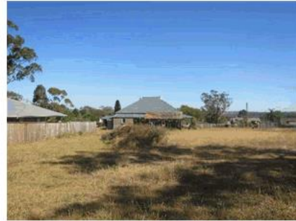
Figure 16: The south-eastern façade of the building, showing the remnant garage structure.
