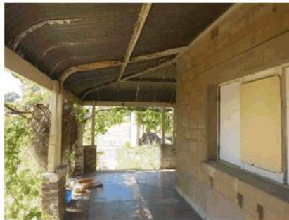
Figure 33: The north-eastern portion of the verandah, facing south-east towards the garage.
