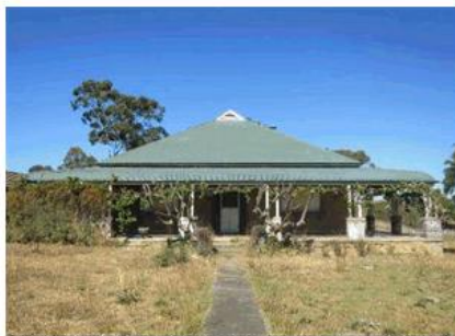
Figure 23: The front façade of Woodcrest from the entrance gate to the property, facing south-west.
