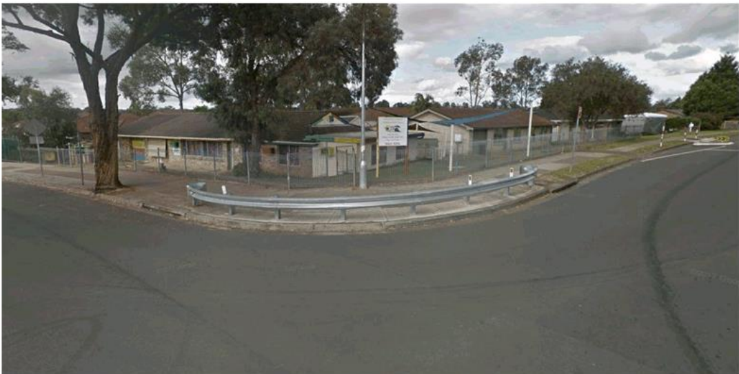
Above: Image of existing barrier facing south east - Source: https://www.google.com.au
