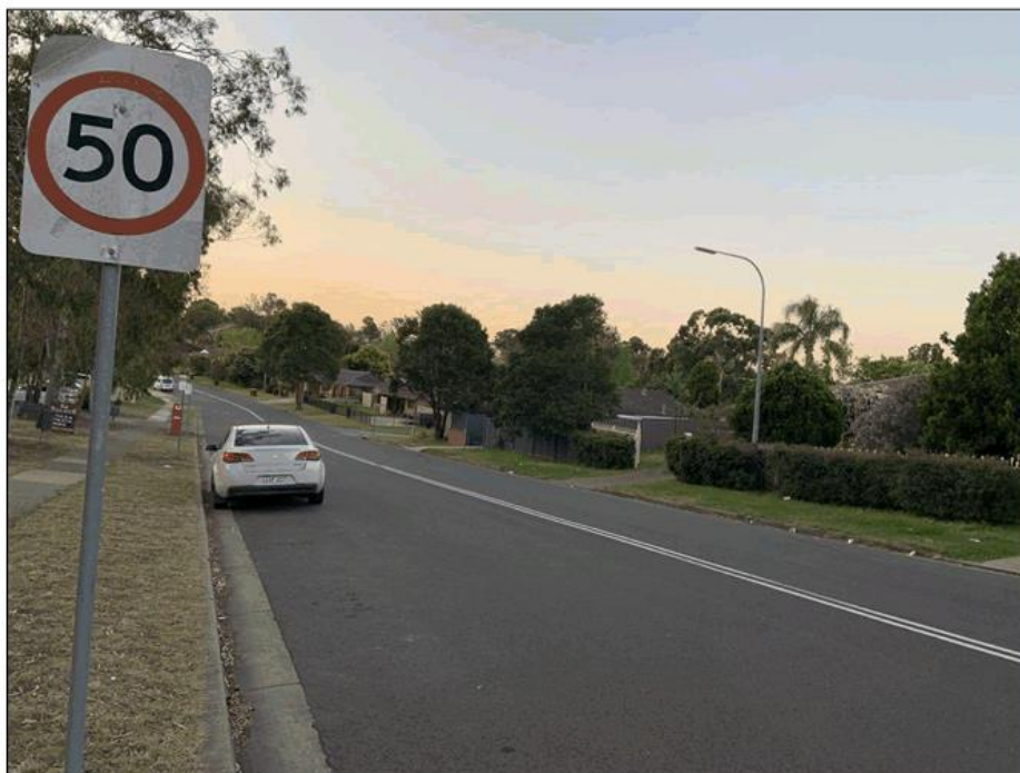
Figure 4b: Hurricane Drive looking north from Kittyhawk Crescent
