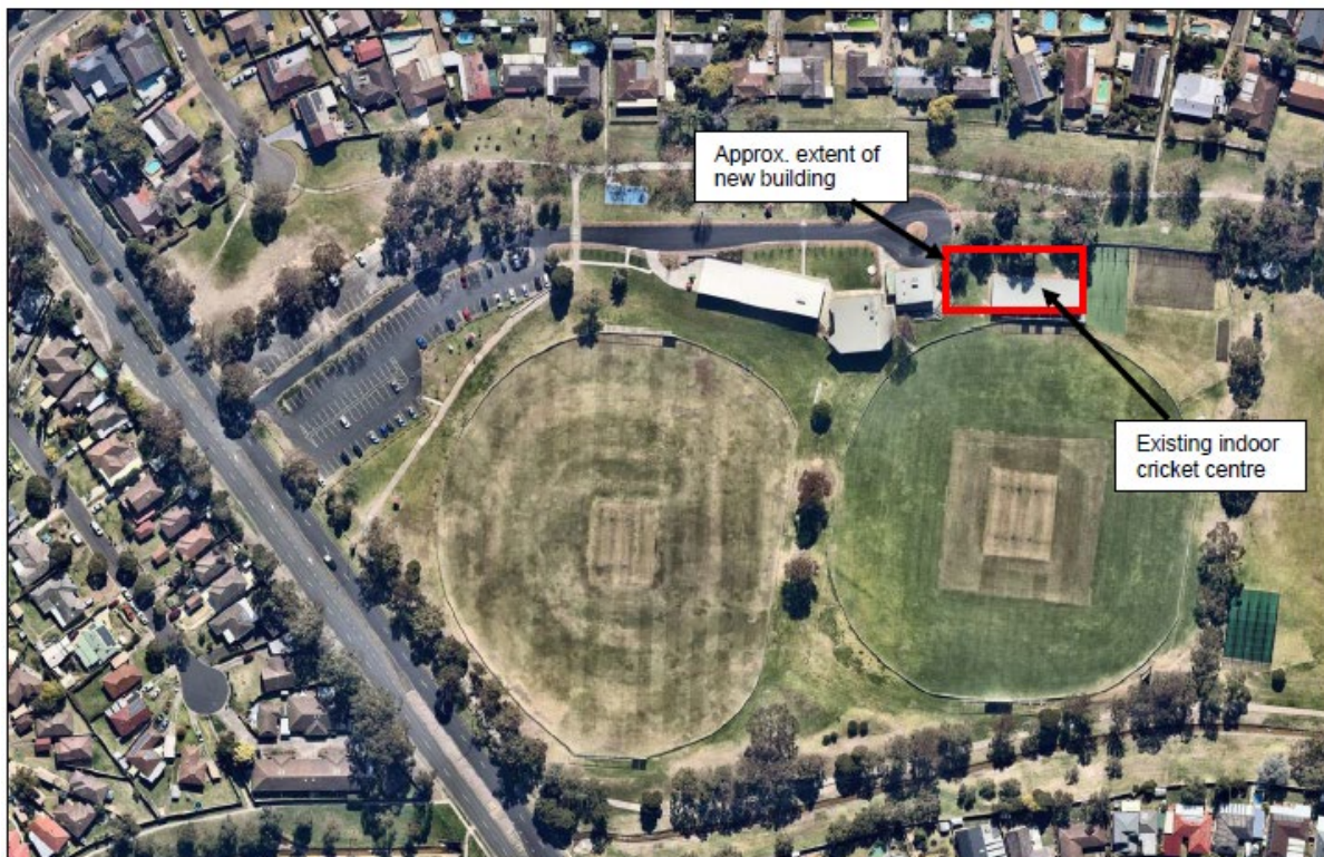
Aerial photograph of the subject site and surrounding locality
