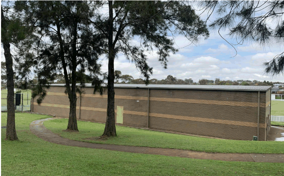
Figure 3 Existing indoor cricket centre – northern elevation
