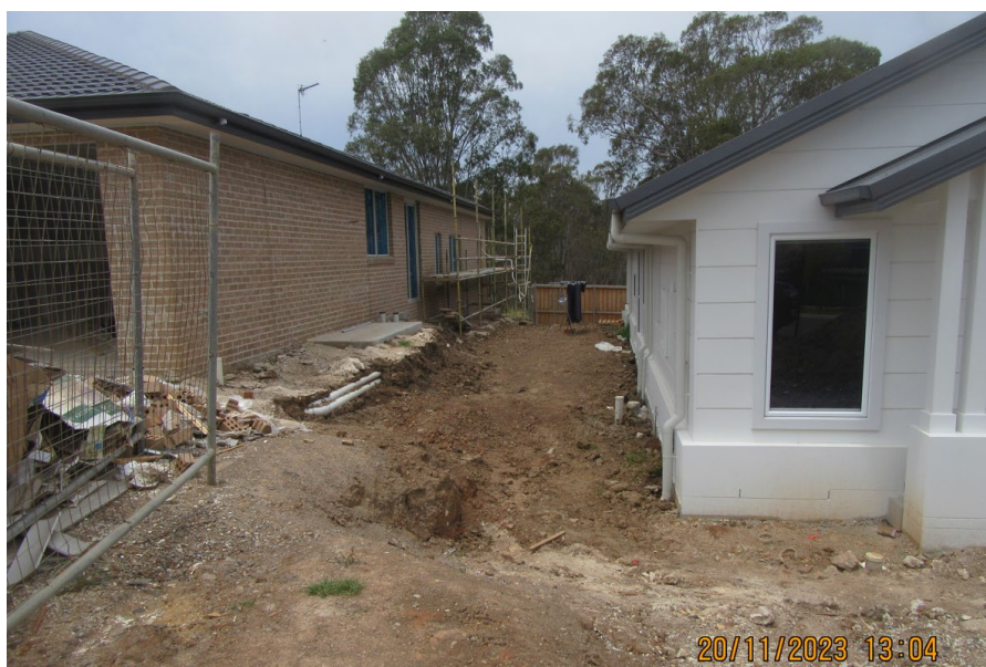
Figure 3 – Site condition between 23 and 25 Roald Place, Leumeah on 20 November 2023
