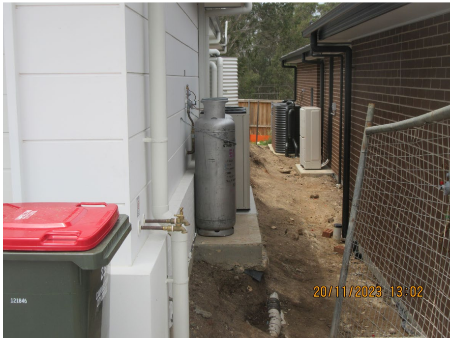
Figure 3 – Site condition between 25 and 27 Roald Place, Leumeah on 20 November 2023
