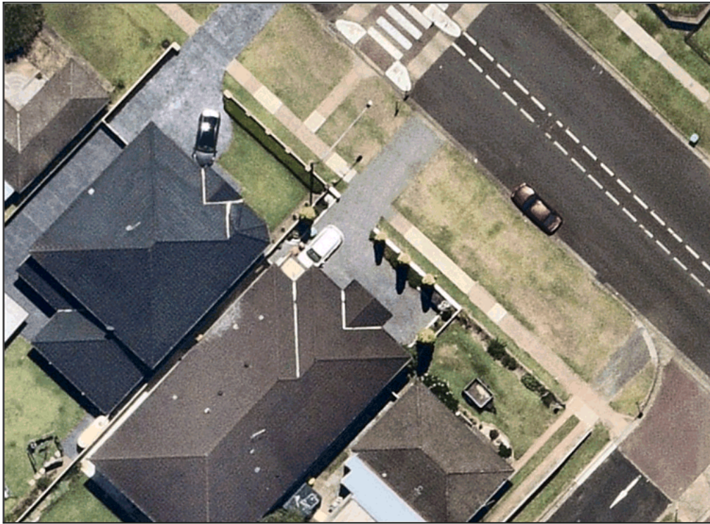
Figure 3: Extract from an aerial photograph which shows that recent development adjoining the Site has significantly more than 30% impervious area forward of the building line.
