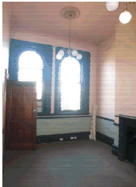
Figure 26 – Original windows and skirting in G.03, bank manager's office. NBRSArchitecture February 2017.
