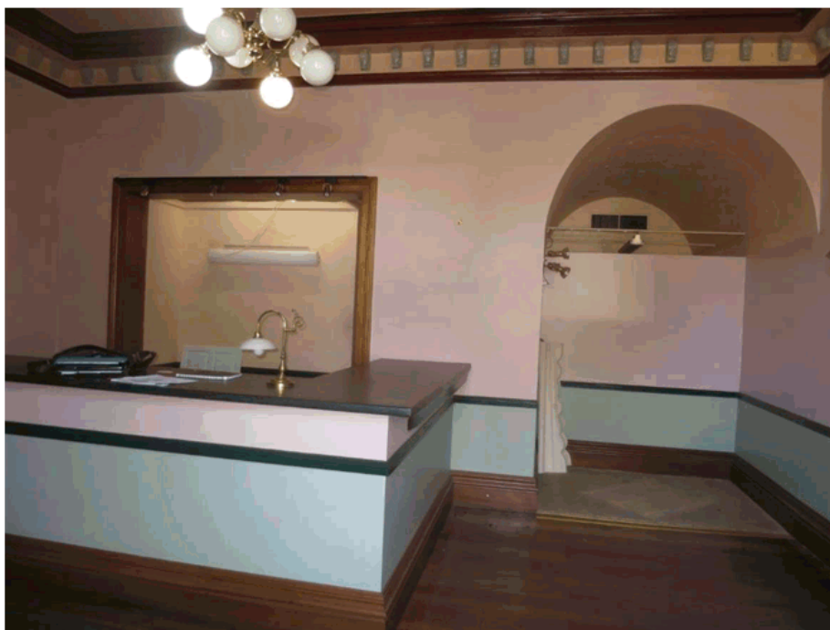
Figure 24 – The banking chamber G.02 showing the recent desk, openings to G.05 and G.06 (former strong room on the right). the skirting is reconstructed, but appropriate. NBRSArchitecture February 2017.
