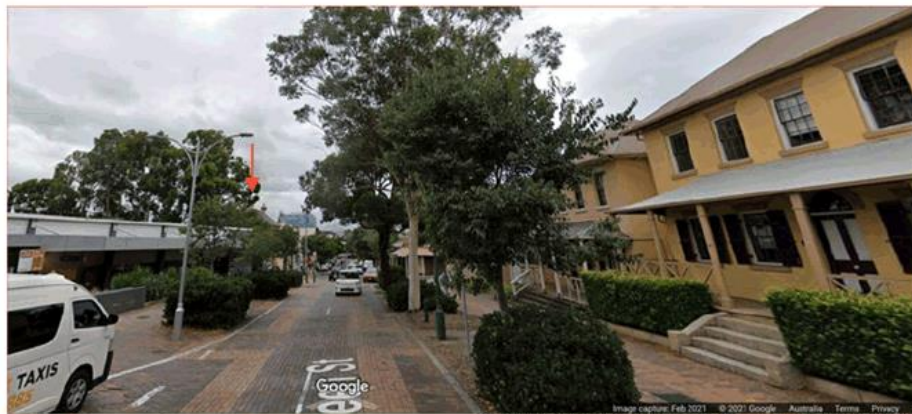
Figure 40 - View north east from the Queen Street conservation area, the red arrow indicates the proximity of the former Bank Building set below the HCA due to the sloping topography. Source: Google Streetview.
