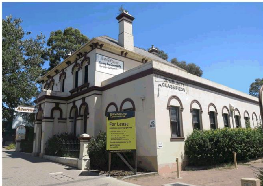
Figure 22 – Southerly view showing the non-significant single-storey extension in the foreground that should be removed from the original building. NBRSArchitecture February 2017.
