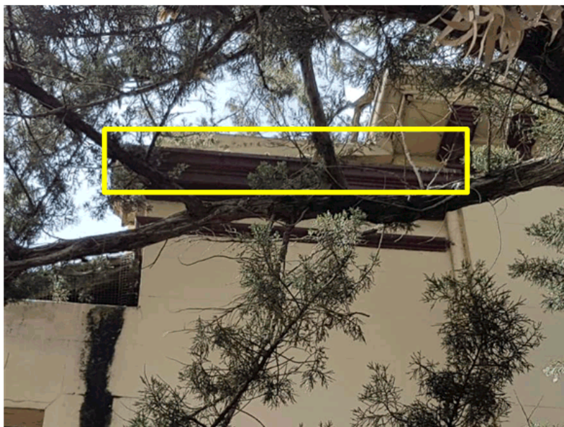
Figure 19 – South West elevation, ground floor - Main Building
