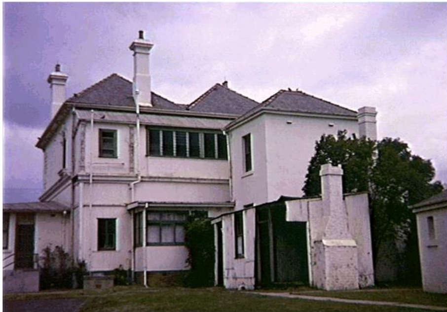
Figure 11 – Rear elevation of CBC, October 1981 / Verlie Fowler. (Source: Campbelltown City Library Local Studies Collection)
