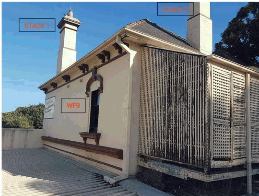
Figure 13 – First floor façade to be retained
