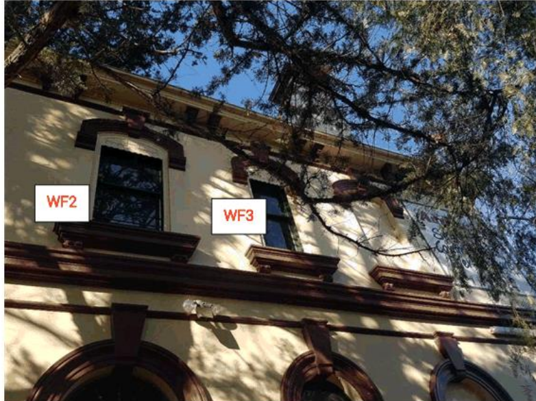
Figure 17 – South West elevation, first floor - Main Building
