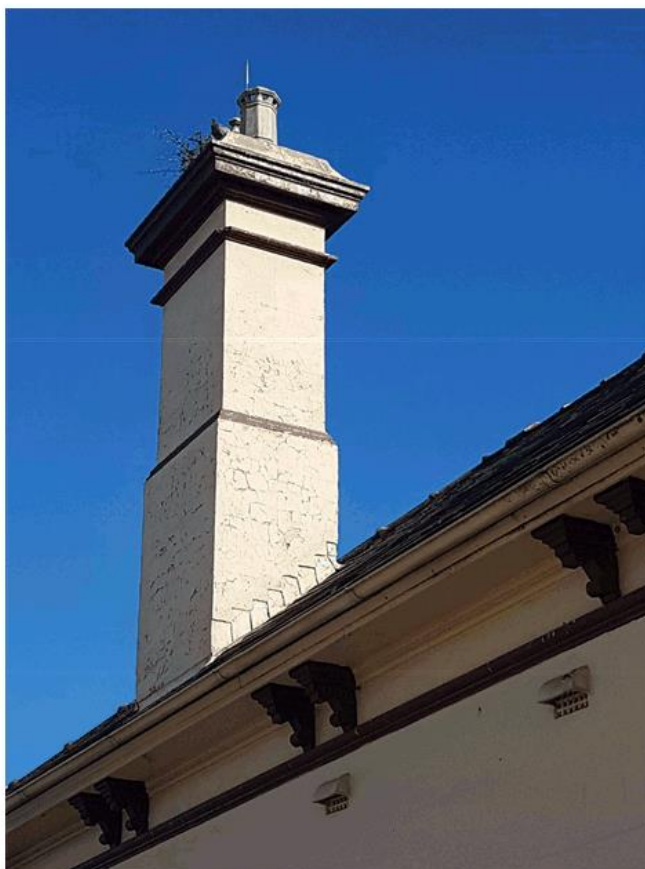
Figure 6 – Chimney Stack 1, North East Elevation, Main Building
