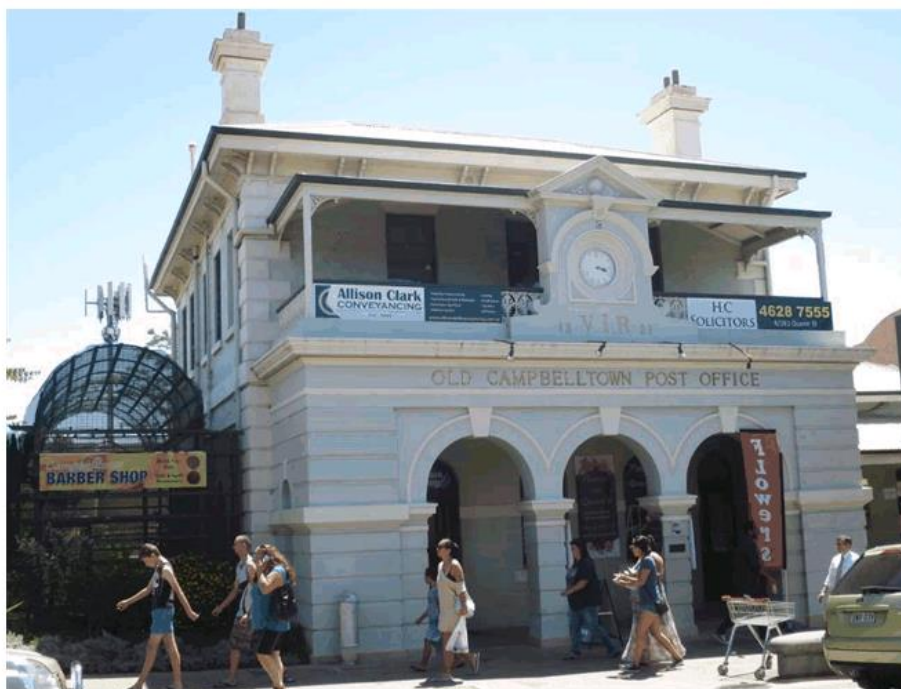
Figure 14 – The former Campbelltown Post Office at 261 Queen Street has a similar scale, form and Victorian Italianate detail as the subject building next door. These two buildings have a visual relationship and contribute to the streetscape.
