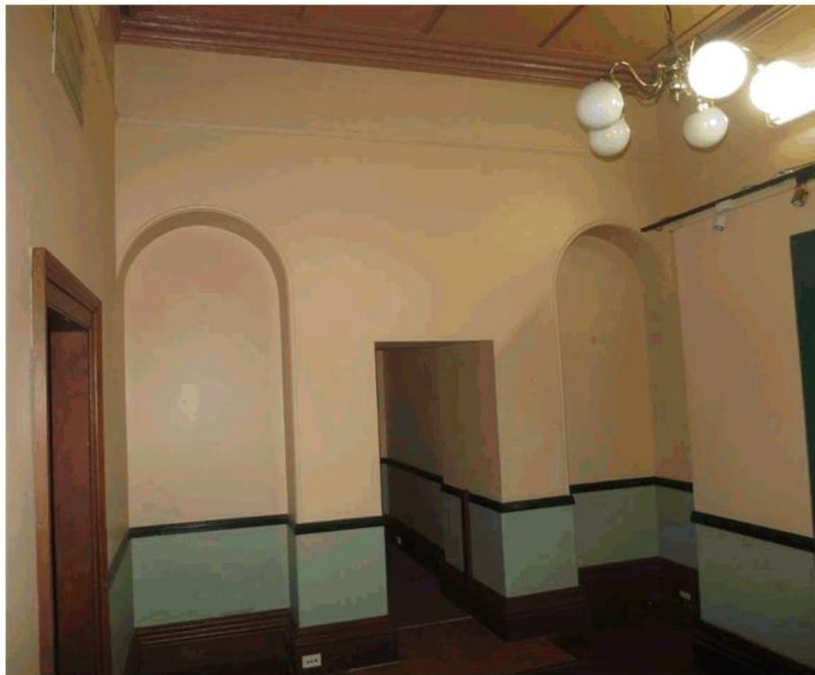
Figure 31 – The original dining room G.05 on the ground floor. The niches, skirting and cornice are original, but the central fireplace has been turned into a doorway to the former strong room. The chimney rises over the left niche.
