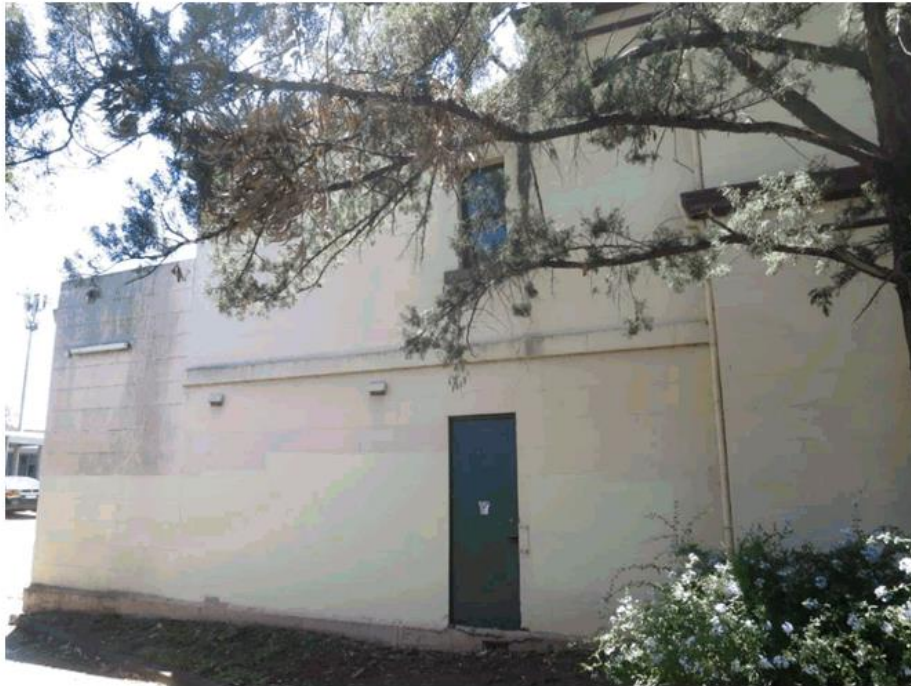
Figure 19 – The south-west elevation of the remains of the service wing. The two-storey section is original but altered. The single-storey section on the left is 1990s fabric on the side of the much longer single-storey service wing that contained the laundry and coal stores. The tree is a Virginian juniper. NBRSArchitecture February 2017.
