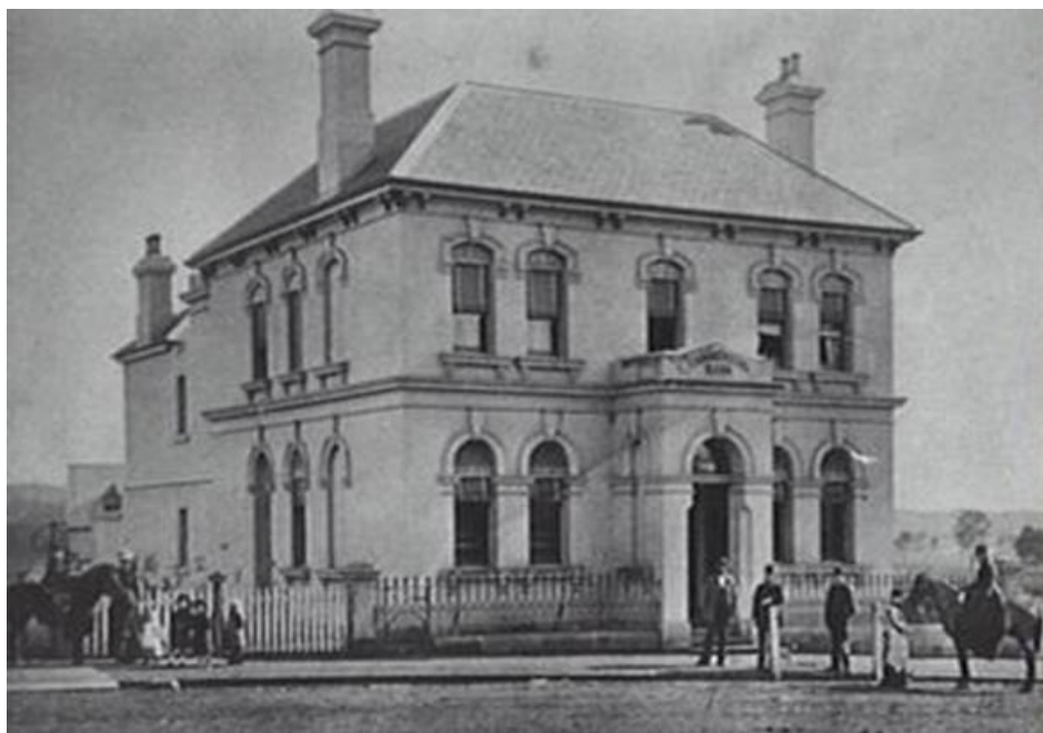
The CBC Bank building in 1881
