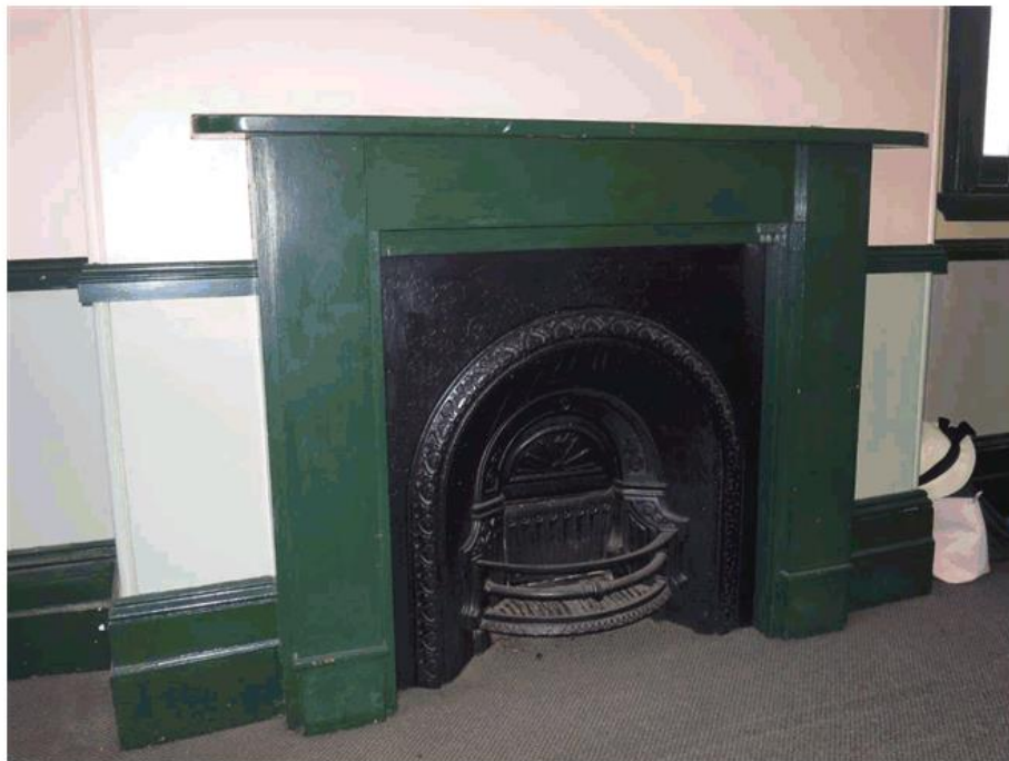
Figure 28 – Likely original cast iron coal grate in G.03. The timber mantelpiece is recent and should be replaced with a Victorian design, preferably in marble. NBRSArchitecture February 2017.
