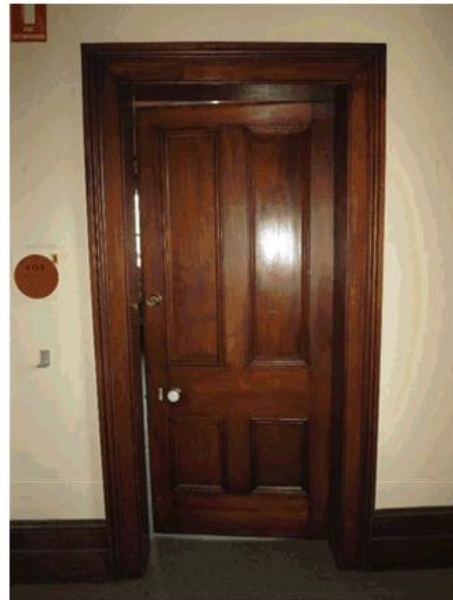
Figure 33 – The intact original door to the former drawing room 1.02. NBRSArchitecture February 2017.
