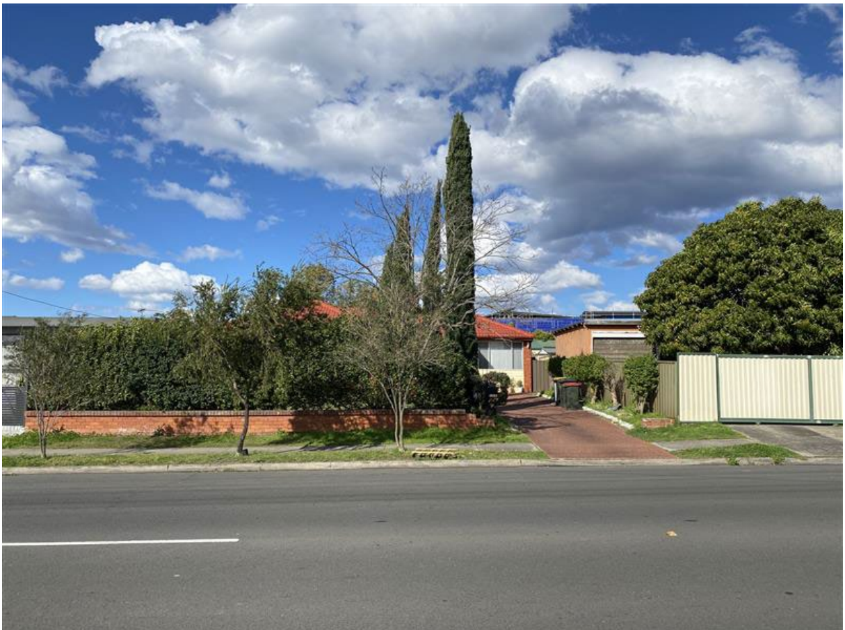
Figure 2 - Current condition of the subject site.
