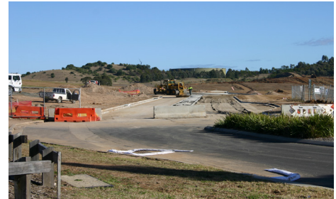
Figure 2.8.2 - Example of residential subdivision under construction.
