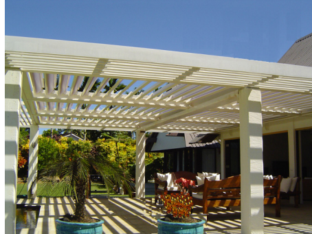
Figure 2.6.2 - An example of a pergola with a zero setback the rear boundary.
