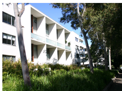
Figure 4.3.2 The provision of deep soil planting can aid the aesthetics of the development.
