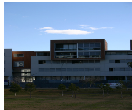
Figure 4.2.1 Example of contemporary residential flat building.
