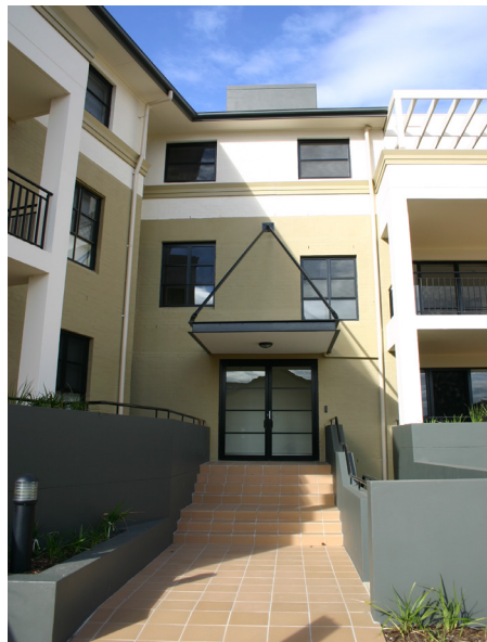
Figure 4.3.1 - Entry to residential flat building.
