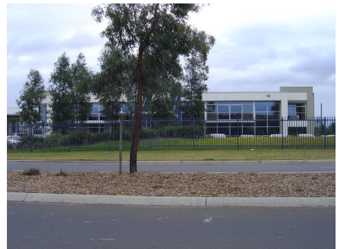
Figure 6.3.2 Examples of loading bays provided for individual units and separate from car parking and landscaped areas.
