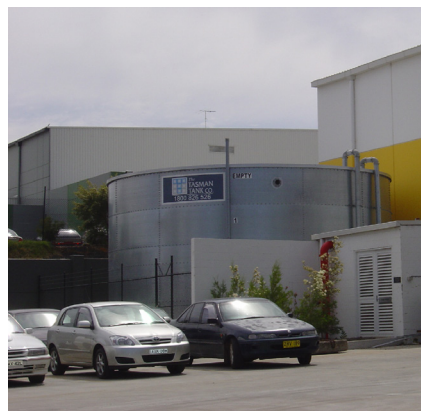
Figure 6.7.1 - An example of liquid storage tank.
