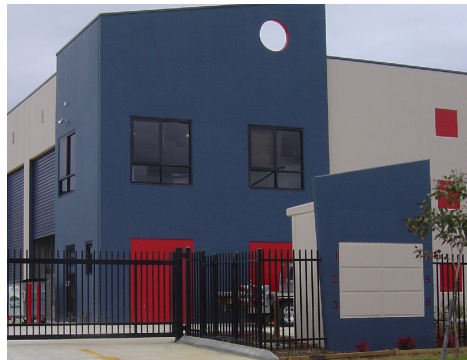
Figure 6.2.4 An example of the use of a palisade fence in an industrial development.
