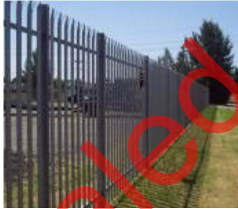
Figure 6.3.5: Palisade fencing.
