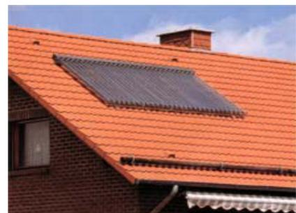
Figure 2.4.2 - Solar hot water panels facing north.
