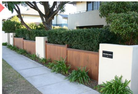
Figure 2.12.1 - Example of a part masonry/part timber fence that helps to define private space and adds interest to the character of the streetscape.
