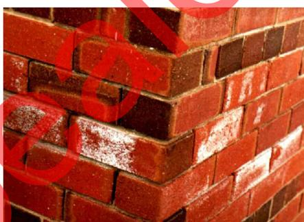
Figure 2.14.1 - Salt damage in the brickwork of surrounding properties identifies a possible salinity problem in the area.
