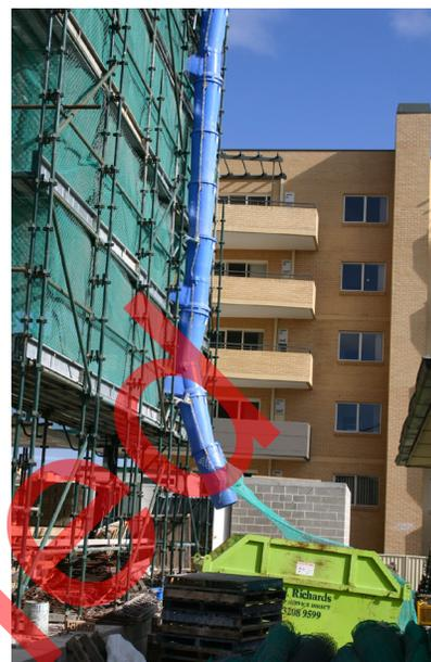
Figure 2.15.2 - Example of management of construction waste.
