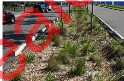
Figure 2.10.1 - Example of a WSUD approach to water quality.
