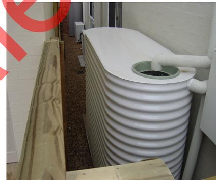
Figure 2.4.1 - An example of a domestic rainwater tank.
