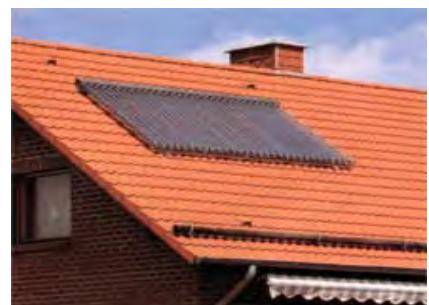
Figure 2.4.2 - Solar hot water panels facing north.
