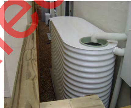
Figure 2.4.1 - An example of a domestic rainwater tank.
