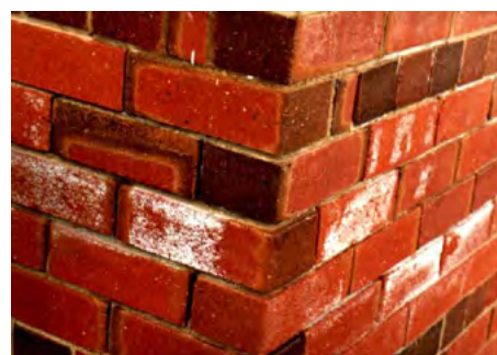
Figure 2.14.1 - Salt damage in the brickwork of buildings identifies a possible salinity problem in the area.
