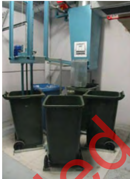
Figure 5.4.5 - Example of waste chute within a residential flat building.
