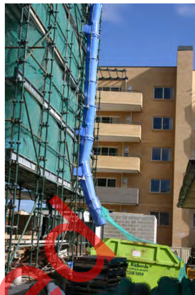
Figure 2.15.1 - Example of management of construction waste.
