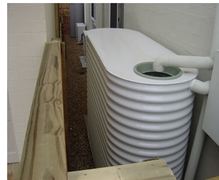
Figure 2.4.1 - An example of a domestic rainwater tank.
