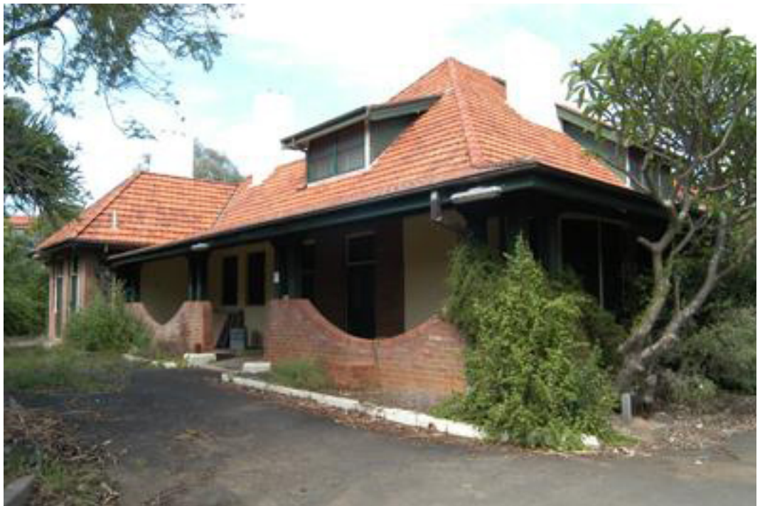
Figure 4.4.1 - A photo of Raith Heritage Item
