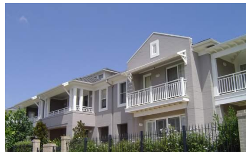
Terrace Style Parking from rear Low fence & landscape to street
