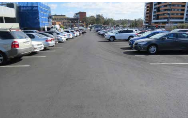
Broughton Street Car Park after Heavy Patching and Microsurfacing
