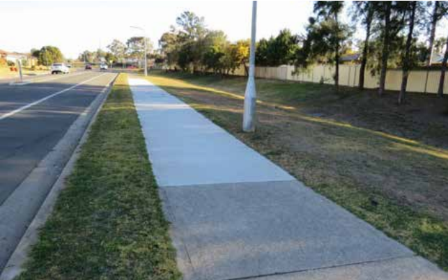
Reconstructed footpath at Copperfield Drive, Ambarvale
