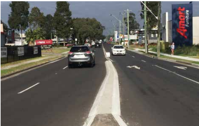
Blaxland Road, Campbelltown after asphalt resheeting
