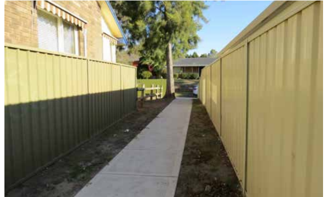
Reconstructed footpath off Donaldson Street, Bradbury
