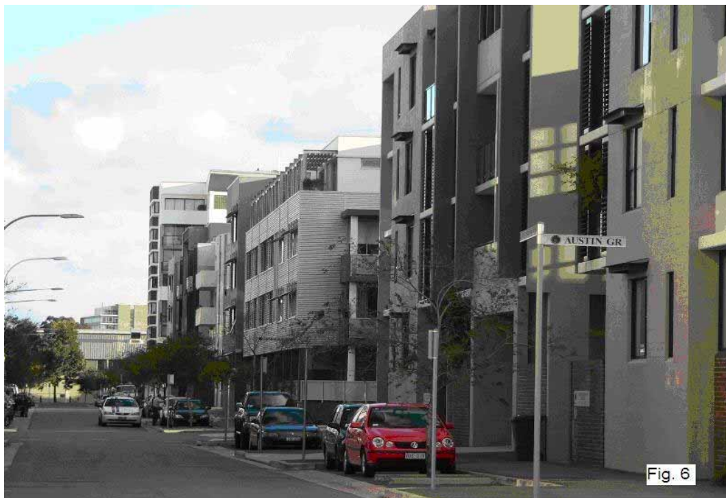
Photograph illustrating small sites, which promote a variation in built form, height and appearance.
