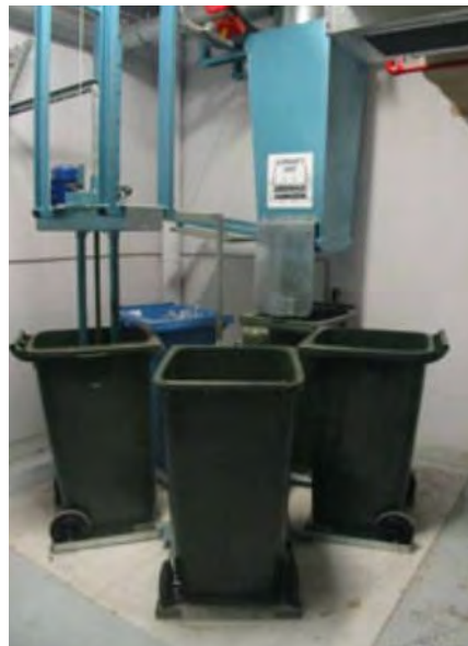
Figure 5.4.9 Example of waste chute within a residential apartment building.
