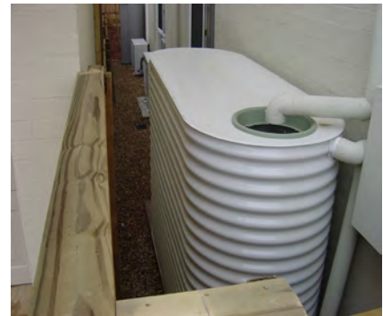
Figure 2.4.1 - An example of a domestic rainwater tank.
