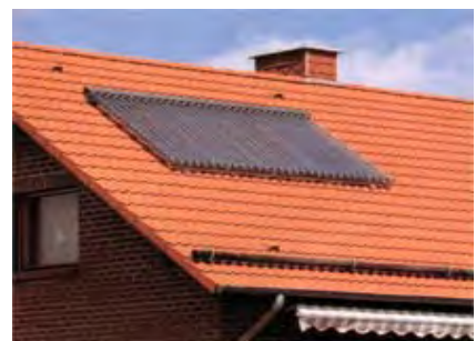
Figure 2.4.2 - Solar hot water panels facing north.
