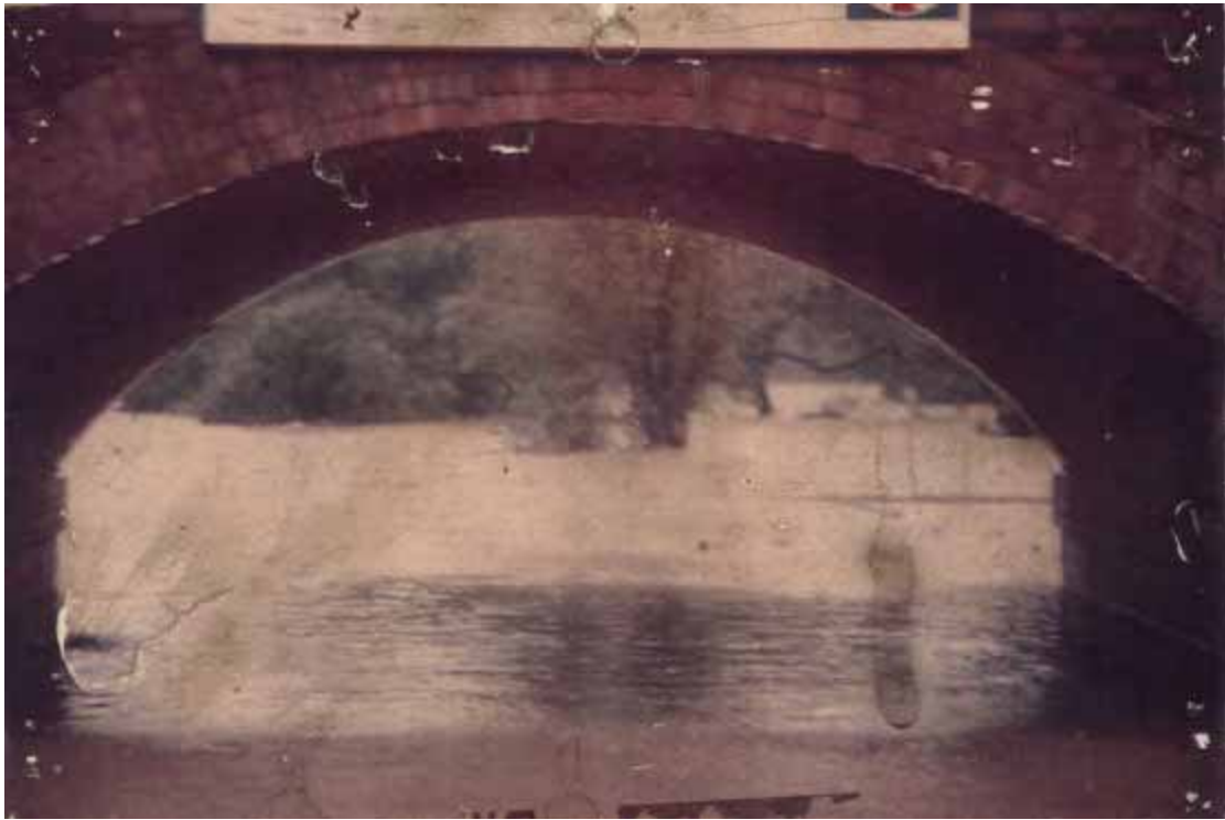
Photo 1 - Flooding under railway bridge at Woodbrook Rd (1986 or 1988 flood)
