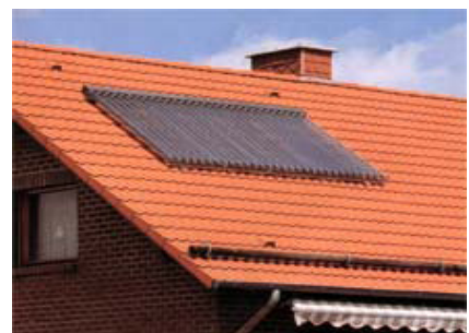
Figure 2.4.2 - Solar hot water panels facing north.
