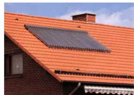
Figure 2.4.2 - Solar hot water panels facing north.
