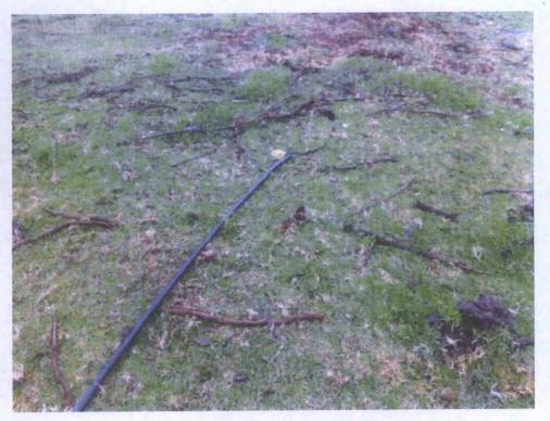
Photograph B16 Lawn sprinkler attached to effluent hose from septic tank.
