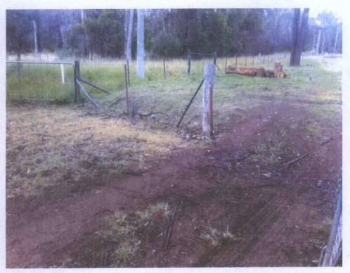
**Photograph B3** Edge of fill layer, near north-eastern site boundary, showing raised ground level due to filling.
