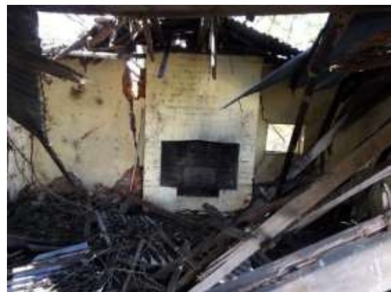
Figure 78: Former gatelodge interior. Roof has collapsed and structure unsound.
