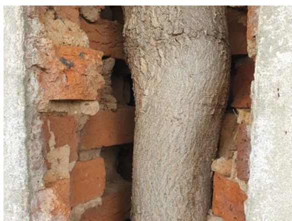
Figure 2.14: View of brickwork of the former gatehouse where a tree has grown through the east wall. Casey & Lowe 2020.
