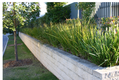
Figure 2.12.1 - Example of a retaining wall.
