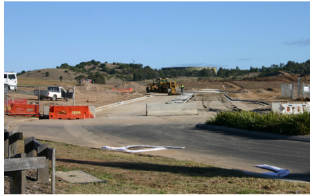
Figure 3.8.2 - Example of residential subdivision under construction.
