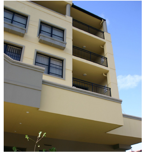
Figure 5.6.1 - Example of mixed-use development.
