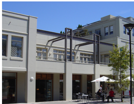
Figure 5.7.1 - Example of mixed-use development.
