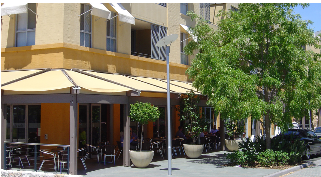
Figure 6.2.2 - An example of a mixed use development within a neighbourhood centre with an active street frontage.
