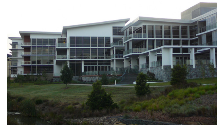
Figure 6.4.1.1 An example of a well articulated commercial building.
