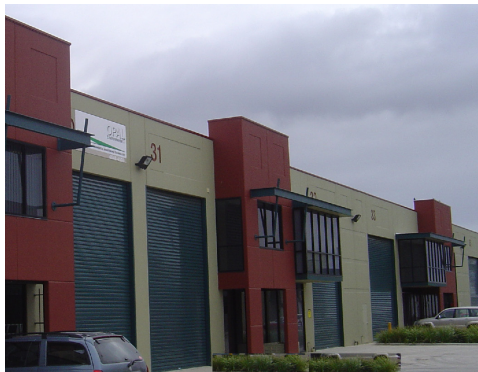
Figure 7.9.1 - An example of a multi-unit complex with individual loading/parking for each unit.
