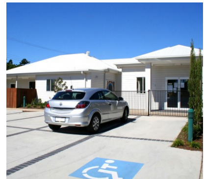
Figure 8.4.1 - Stacked configuration of car parking spaces as shown in this photos will not be included in the parking calculations.
