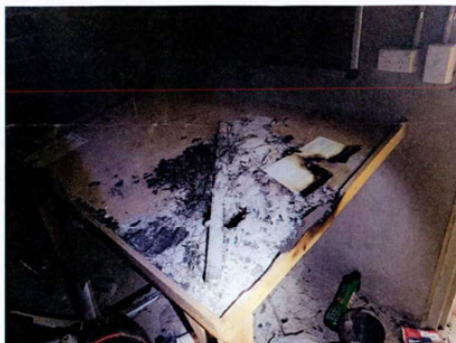
Image 1: Evidence of previous fires in the fire control room.
