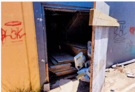
Image 4: Blocked fire exit.
